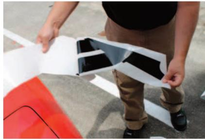
2. Spray the work area with application fluid (4 drops detergent to 1 pint of water), then separate the decal from the paper and spray the back (tacky side) of the decal.
